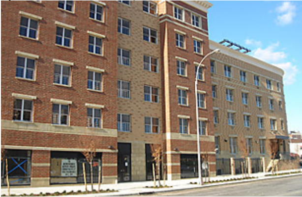
Intervale Green, an environmentally friendly housing development for low income families in the Bronx, New York. Whedco
