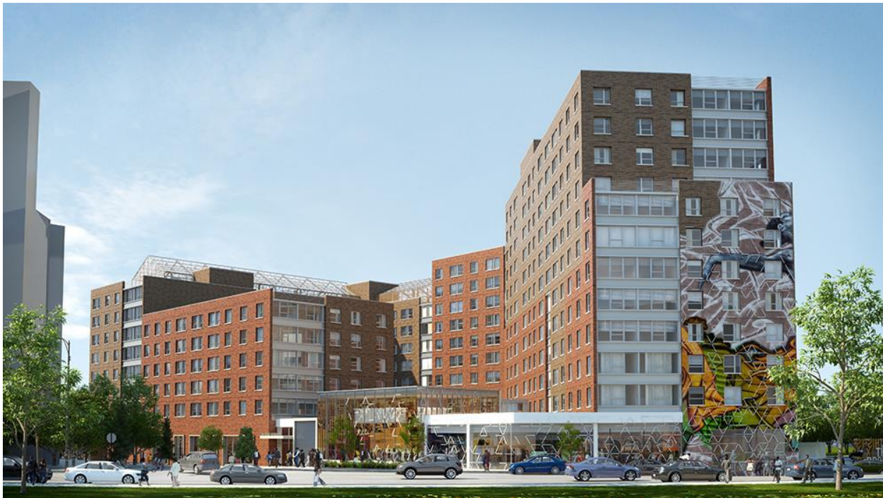
Bronx Commons, bringing 303 affordable apartments to Melrose
