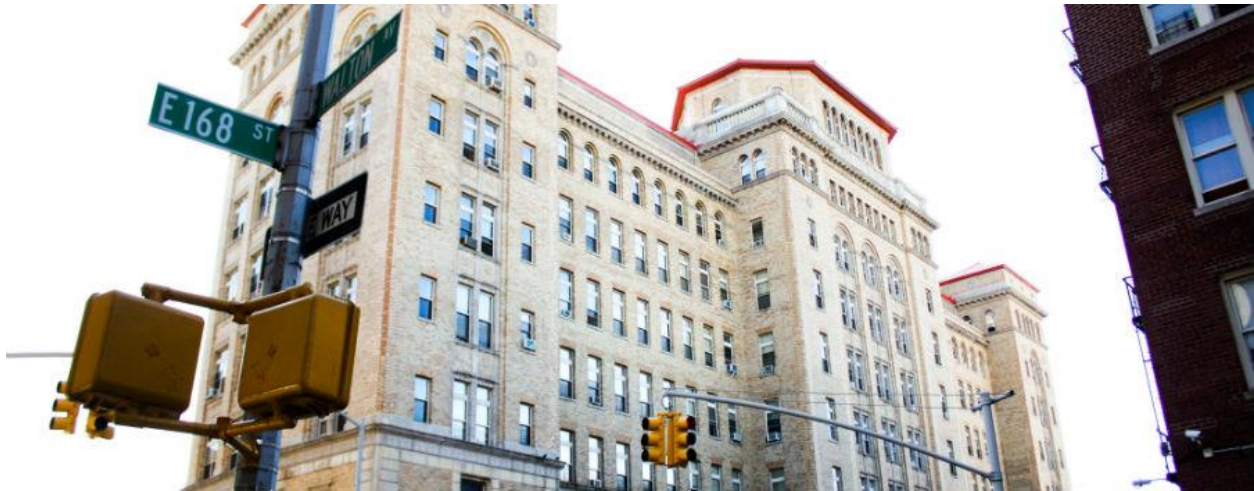
Urban Horizons/former Morrisania Hospital, photo by Samir Abady
