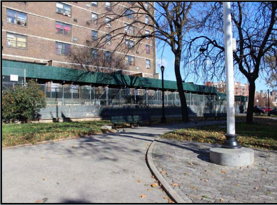
Railroad Park on E. 161st Street
