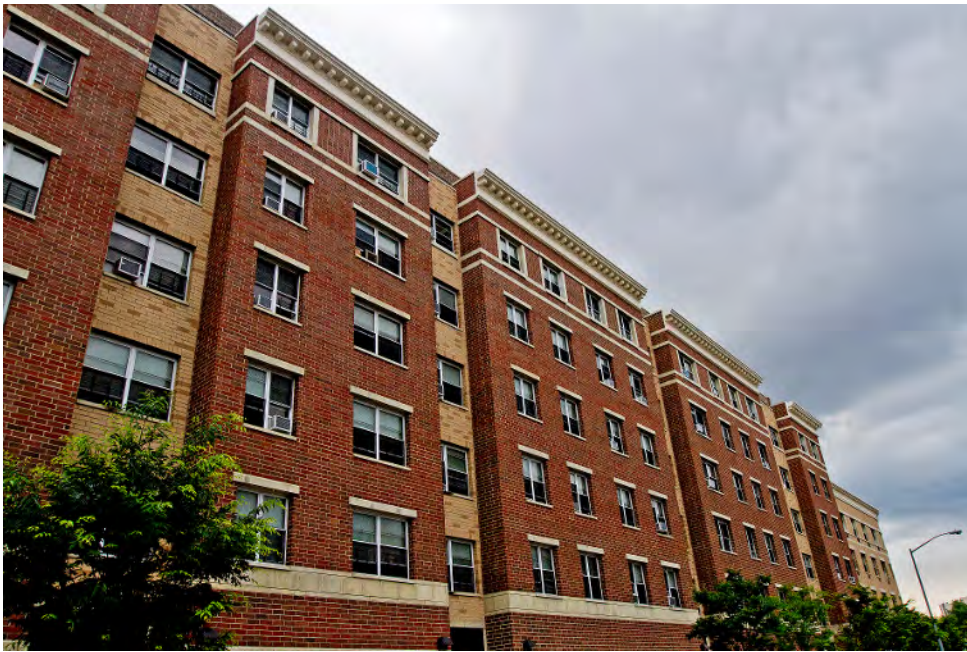
WHEDco provides homes for 800+ people in two affordable housing developments in the South Bronx, Urban Horizons and Intervale Green (pictured above), with a third building under construction.
