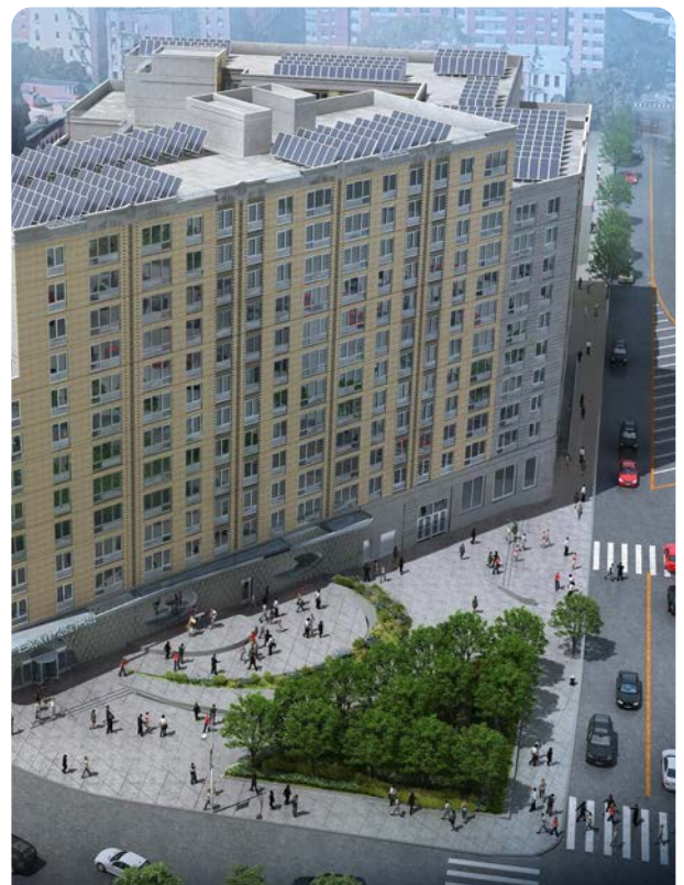
Rendering of Bronx Commons, WHEDco's third affordable housing development, currently under construction. Completion is expected in the fall of 2019.
